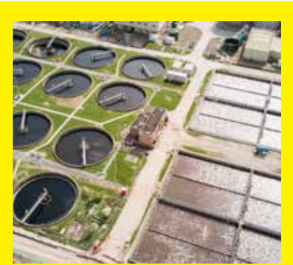
Water Treatment Works
